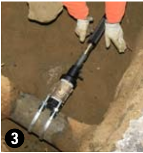
3 Turn independent feed until the pilot drill touches the pipe.
