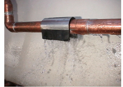
Loosen the bolt and separate the two parts of the clamp. Snap top half of clamp with rubber directly over leak ensuring the thin part of the gasket is over the fitting and the thick part is over the pipe.
