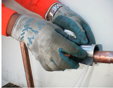
Loosen the bolt and separate the two parts of the clamp. Snap top half of clamp with rubber directly over leak ensuring the thin part of the gasket is over the fitting and the thick part is over the pipe.
