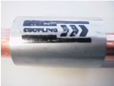
With arrows facing the solder joint, slide over until flush with coupling.
