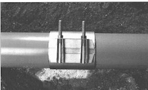
Completed JCM 168 Clamp Installation
